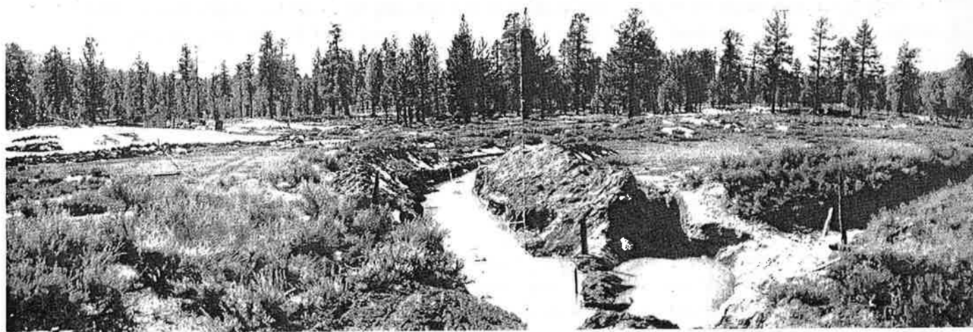
Figure 63. Panorama of Upper Holcomb Valley gold placer area, east part of the Slap Jack claim. Camera facing south; February 1940. Tailing pile, left middleground, at Plant No. 1 of Holcomb Valley Placer Company. Ditch, in foreground, for water development, is in Recent alluvium and gravels locally termed "meadow ground". The gold-bearing gravels that were mined, included in the older alluvium and gravels shown on plate 1 and locally termed "bench gravels", occupy the gently rolling topography in the background, commencing at about the tree line. Photo courtesy Lacy Oil Tool Company, Los Angeles, California.
